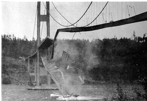
1940, Tacoma Narrows Bridge
